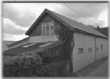
The Brick Barn, EX4 2JH
